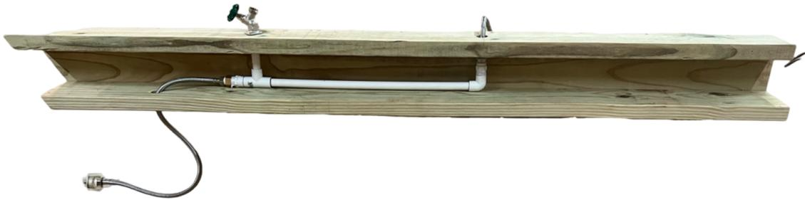
*Note: Once the pipe with primer and glue is inserted into the PVC tee you won't be able to twist it, so make sure to orientate the spigot matching up the two screw holes in the spigot to the two predrilled holes through the enclosure.*
